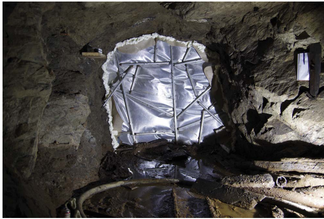
FIG. 11. The “Quick-Erect Stopping System” (QESS) set up in the Querschlag 60 gallery in Schneeberg to shut off the radon rich Querschlag 60 from the Markus Semmler gallery to prevent the miners from radon exposures.
